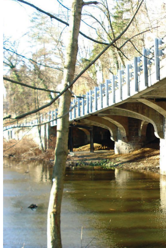
◀ The bridge's concrete-encased brackets and core.
