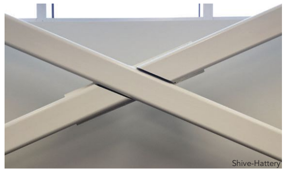
▲ The X-bracing was typically HSS5×5× \frac{3}{8} .
